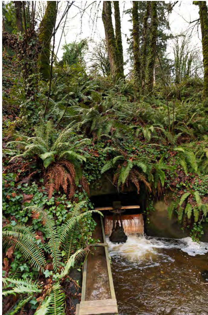
Photo 1. North Creek culvert at Harborview Drive, culvert outlet and water diversion for RSI
