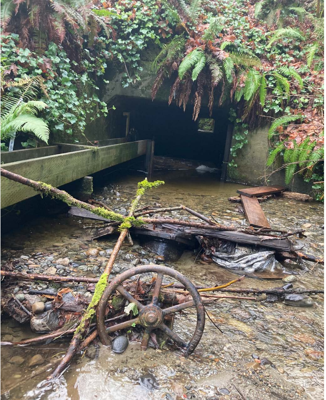
Figure 3 – Fish passage barrier downstream of Phase 1 property – to be replaced with a bridge
