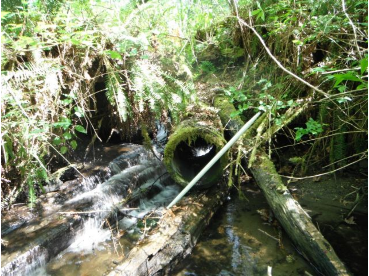
Culvert under former driveway. Driveway and culvert are both washed out and form a partial stream blockage. Photo courtesy WDFW.
